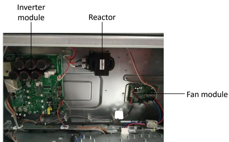
Figure 5-1.3: 18-30HP top layer of electric control box
